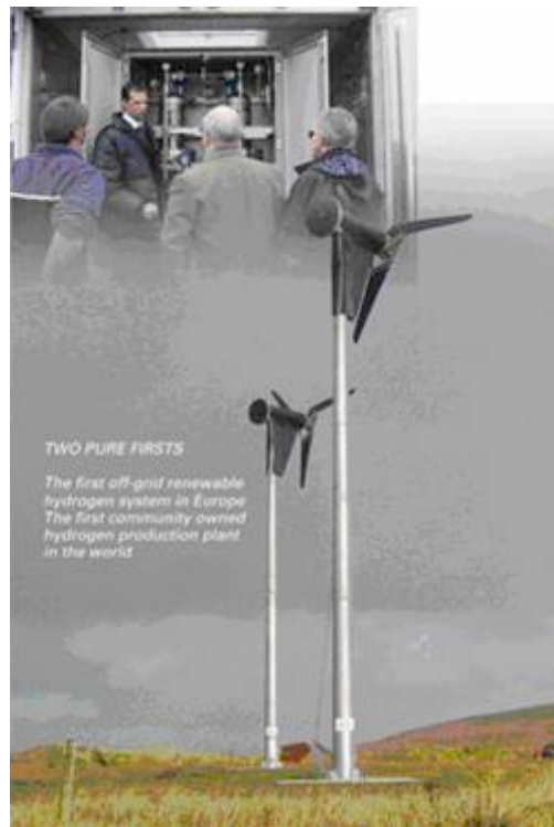
Figure 5.3: The PURE project converts the output from two 15 kW turbines to hydrogen, which is used to run a nearby business facility ( https://pureenergycentre.com/ ).
