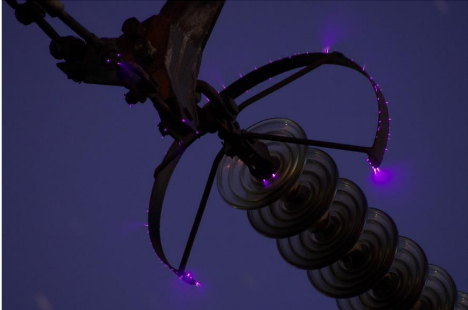
Corona emission from energized parts of a transmission line suspension insulator
