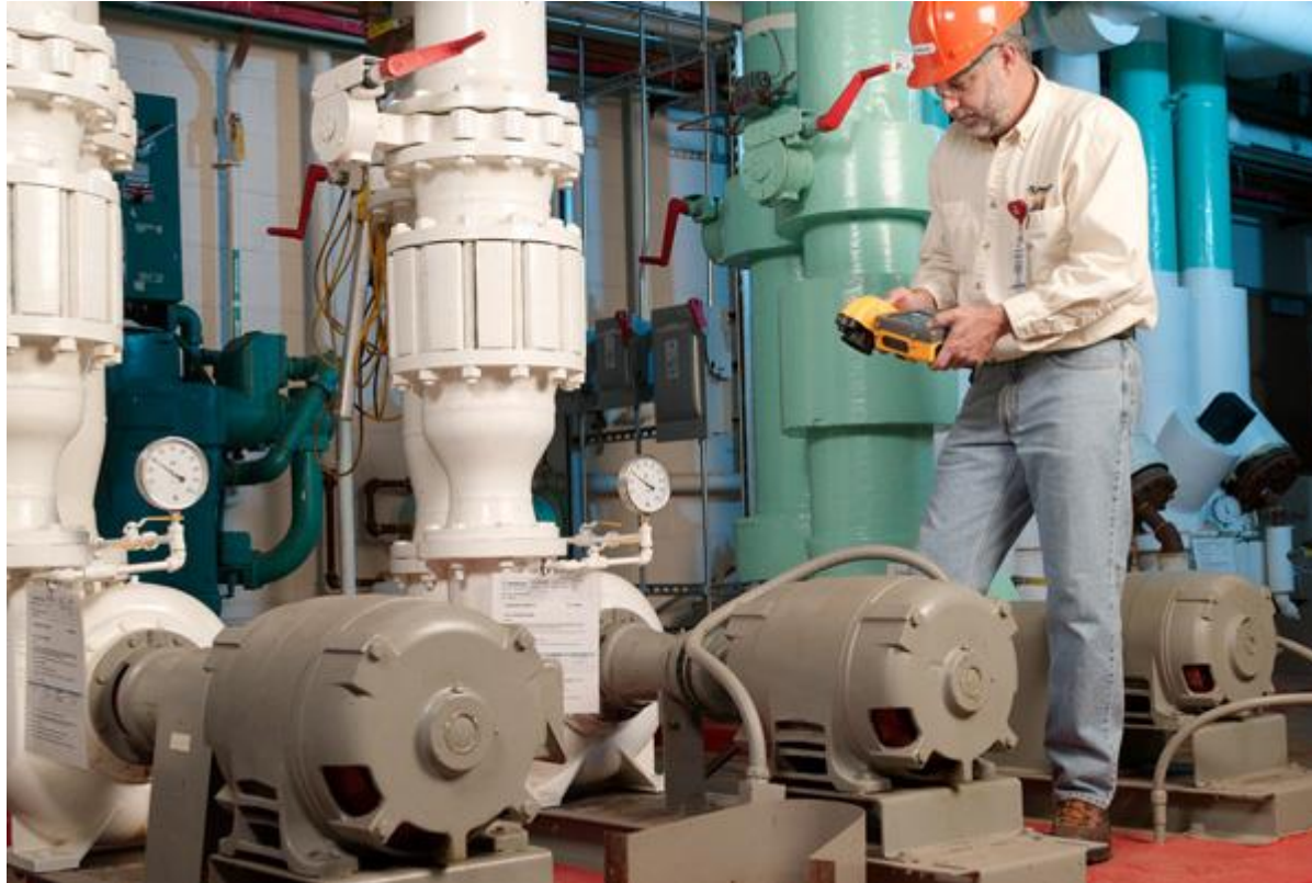
IR Surveillance of Boiler Feed Pump Motor
